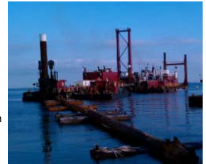
Dredging for Birth 12 begins at Port Manatee
